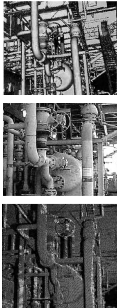
Figure 10. Comparison of images obtained by shrink-wrap laser scanning (top), digital photography (center) and laser scanning (bottom) source: www.wikipedia.org
